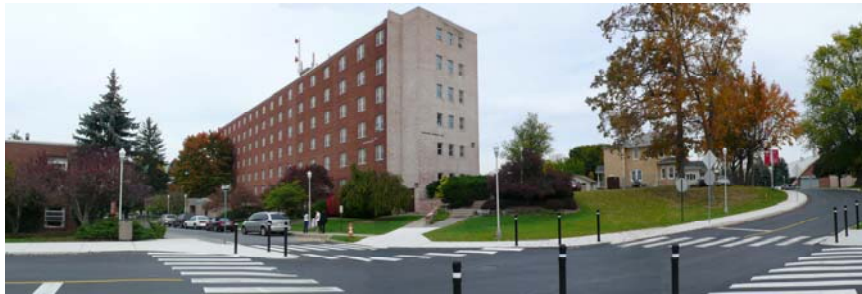
Normal Street – Existing conditions looking north
