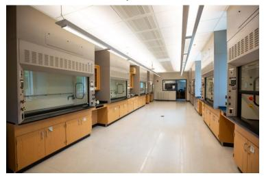
The **chemical fume hoods** used for the general chemistry laboratories are located in Science & Technology Center room 140. The hood room is a highly ventilated, air-controlled facility with 8 class A hoods to contain and remove gases and fumes generated during experiments via an elaborate exhaust system. This supports and is flanked by two general chemistry laboratories. Contact **Dr. Steven Boyer**.
